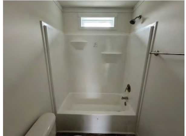
Bath #2 Fiberglass Tub shower
